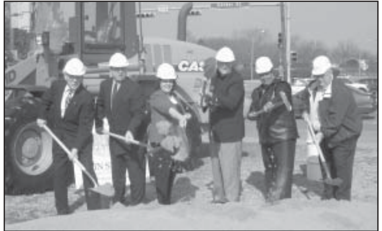
Local elected officials help Monte Anderson break ground at the new Main Station development located at the corner of Main Street and Center Street. Pictured from left to right is Mayor Glenn Repp, project developer Monte Anderson, Councilmember Marilyn Massey, Councilmember David Green, State Representative Yvonne Davis and Councilmember Grady Smithy.
